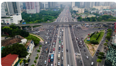
Vietnam metropolis infrastructure in progress.
